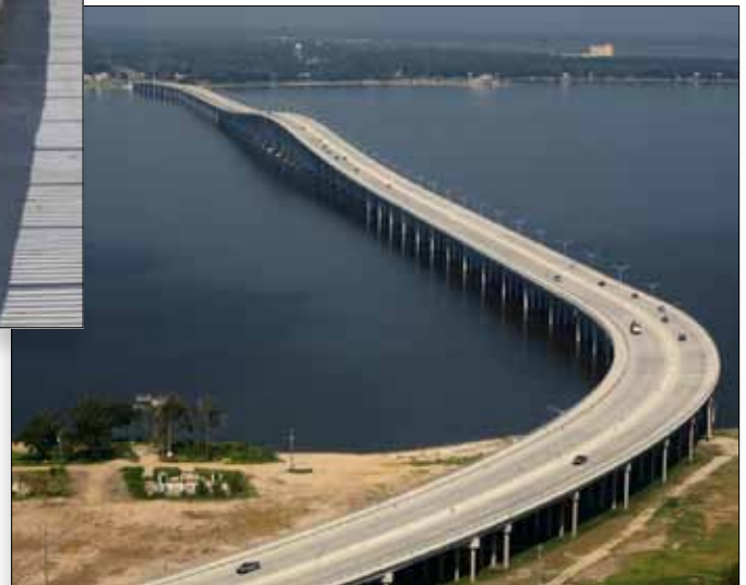
Bay of St. Louis Bridge
